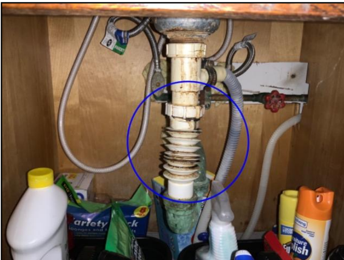
Nonstandard materials and patches
