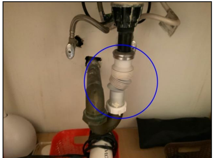
Nonstandard materials and patches
